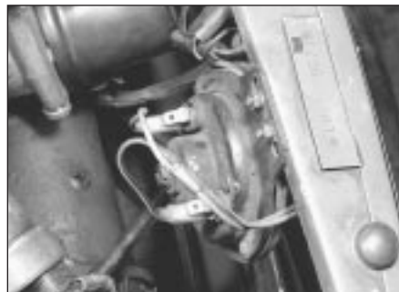
9.1 Horn location showing electrical leads and mounting nuts
