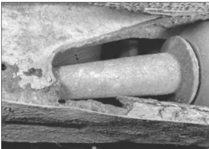
6.3 Advanced state of corrosion on rear subframe side member
